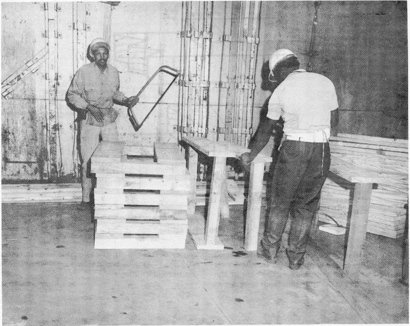
Figure 6-19. Onboard assembly of prefabricated structures.
